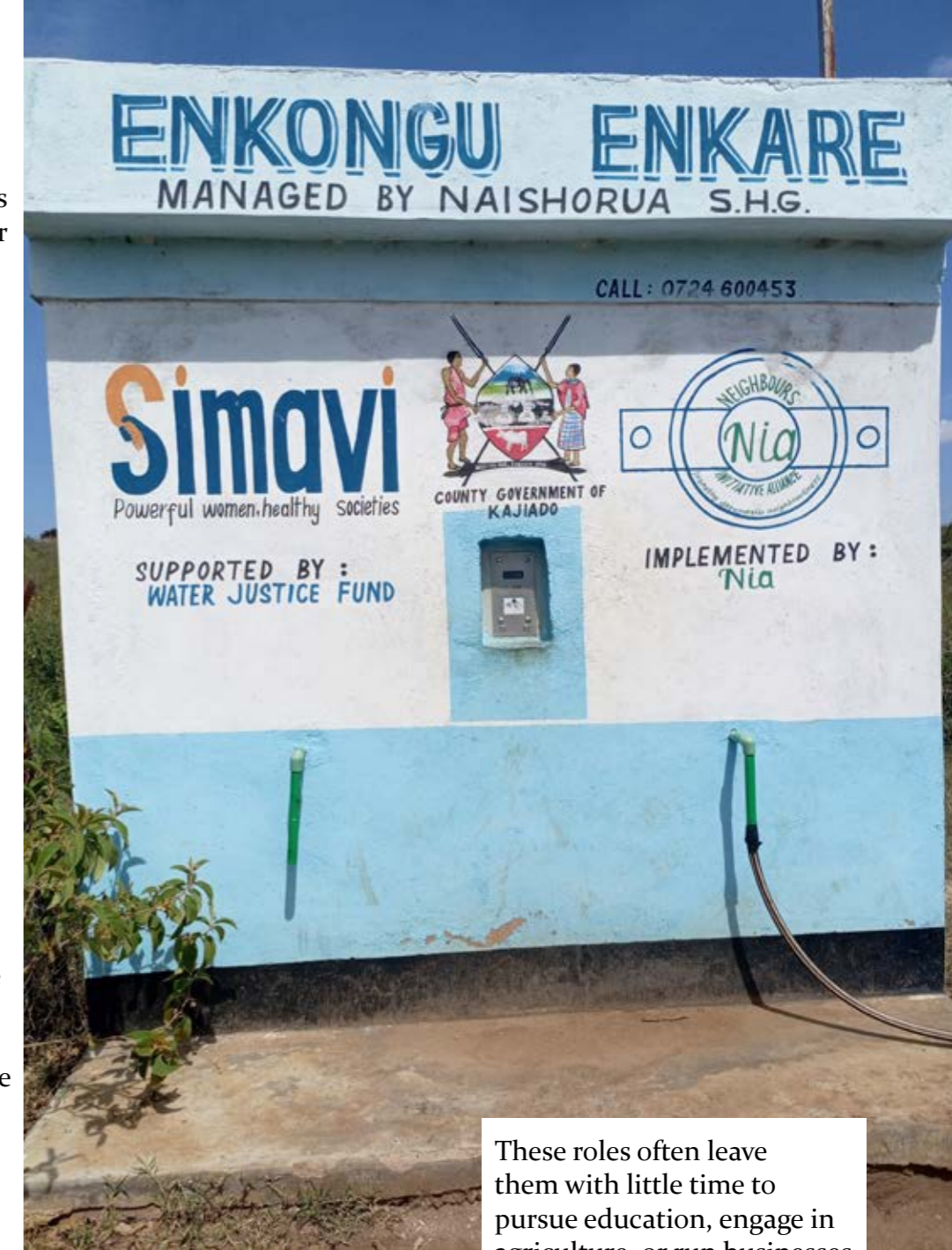
The automated water kiosk managed by the Naishorua Self-Help Group.
